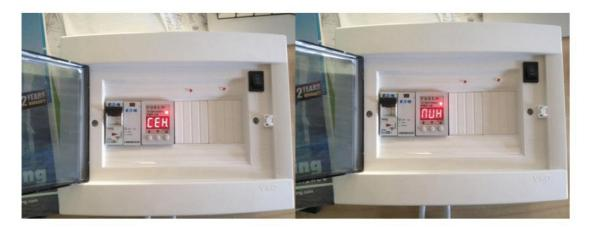
4. Select the t2 (pause time) option and press the "to the side" arrow (button 4) again... Repeat the programming cycle according to point "3" of these instructions. The above programming cycle sets the time pump "pauses".
